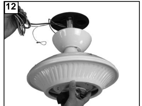
12 Carefully lift fan assembly onto mounting bracket. Rotate fan so that the notch on the ball engages the ridge in the mounting bracket. This will allow hands-free wiring.
